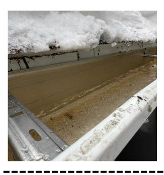
Gutters should always be installed under the drip edge. We returned to this job after leak complaints only to find out the gutter was installed incorrectly. These are service calls that are very easily avoidable if you take your time and do things the correct way.
