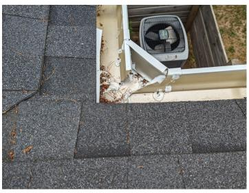
Do NOT leave gutter in miters like this. This will hold water and cause issues. Gutters should be trimmed so water can flow easily.
