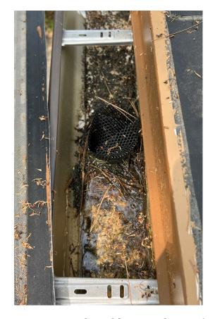
Do NOT ball up basic screen, put it in the downspout hole, and then install Armour Guard over it. We cleaned these gutters for free because of this.
