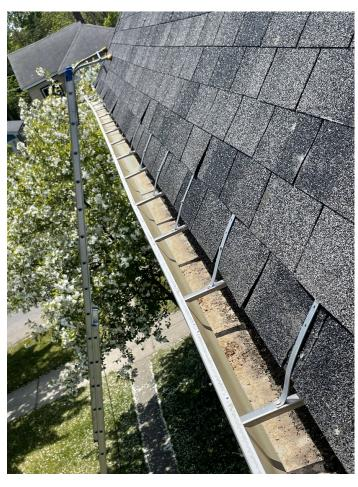
Vampire straps should NEVER be installed like this. They need to go under the first row of shingles. Flat head screws should ALWAYS be used.
