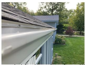
DON'T damage the drip edge and shingles when installing the gutter. This drip edge was installed incorrectly by the roofer (nothing holding the drip edge in place other than the glue used to attach the shingles - yikes!) so it caused it to look super damaged. It is still important to take your time and let the office know when something doesn't look right.
