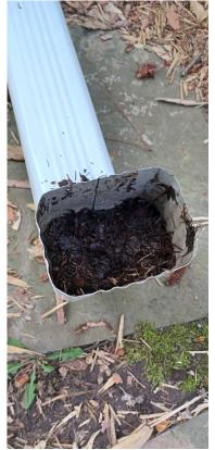
When installing amour guard on existing gutters - you *MUST* clean out the downspouts along with the gutters. We have had to return to cover jobs to unclog DS multiple times now - including this one pictured.
